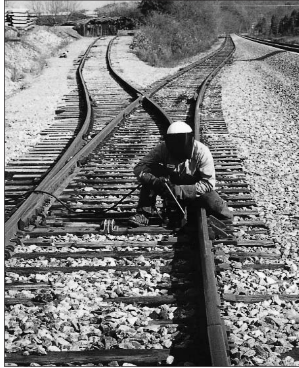
Welding Switch Points
